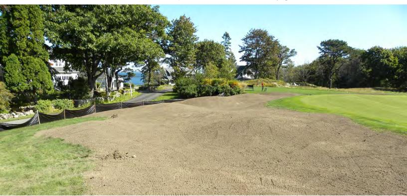
A silt fence prevents stormwater runoff from carrying sediment offsite. © Bob Searle
