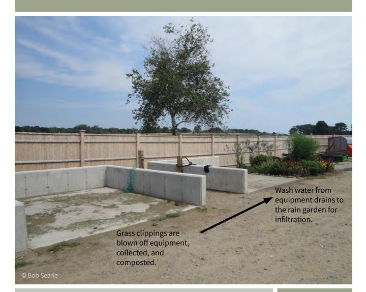
Abenakee Club installed wash pads in 2012 to wash vehicles and equipment. Wash pads allow equipment to be cleaned while protecting the environment from contaminants that would otherwise drain into local water sources or cause stormwater contamination.
